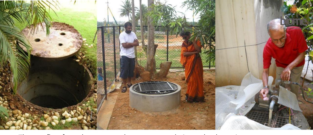
The overflow from the sump, or the stormwater drain, or the downpipes are connected to the well. Wells are also fitted with electric motors. They are covered with a safety grill, or an RCC slab with a manhole or peephole. This helps sunlight enter the open well, creates an access point for maintenance. It also helps us look inside the well and monitor water levels
