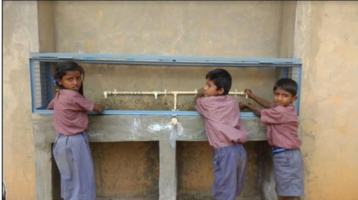
Hand wash was built with a mesh around to prevent incidences of vandalism
