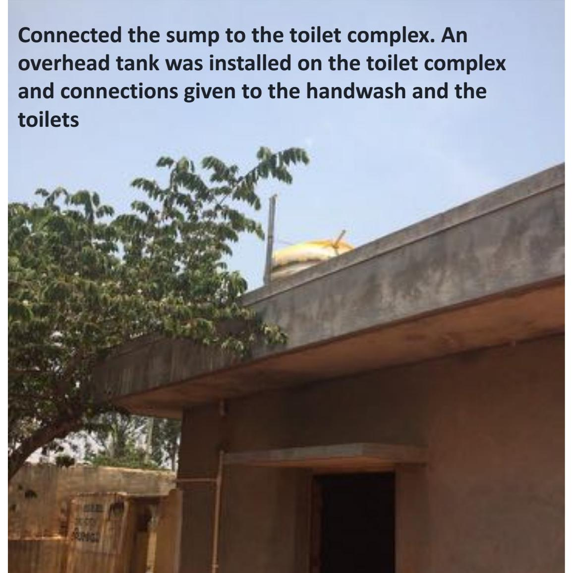
**Connected the sump to the toilet complex. An overhead tank was installed on the toilet complex and connections given to the handwash and the toilets**
