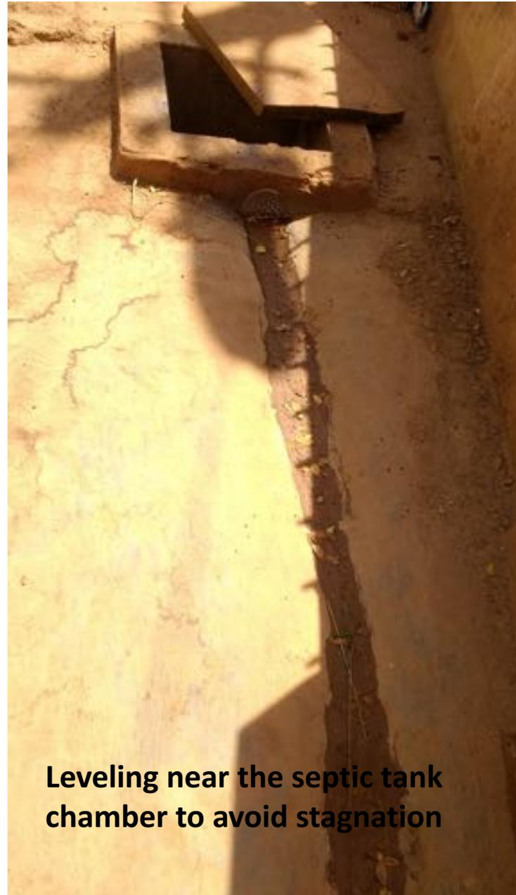
**Leveling near the septic tank chamber to avoid stagnation**
